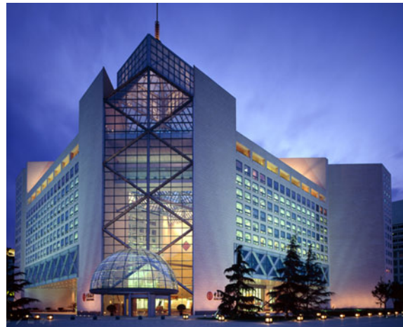
Bank of China HQs, Beijing, China
